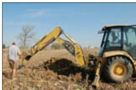
**HUNT AND POKE:** Neither a backhoe nor a tile probe could find the 4-inch-diameter tile running through this field.
